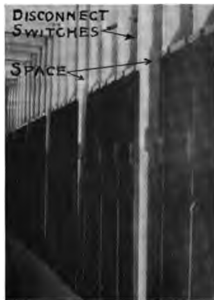
Fig. 2. Separation of High-Tension Bus-Compartment into Circuit-Groups.*
